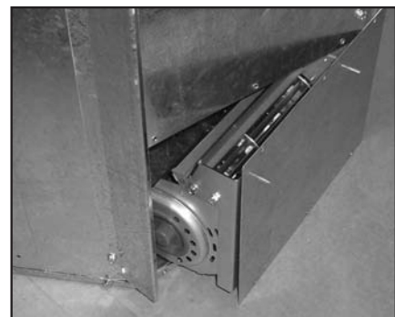
Figure 53: Installing Fan Through the Back.
